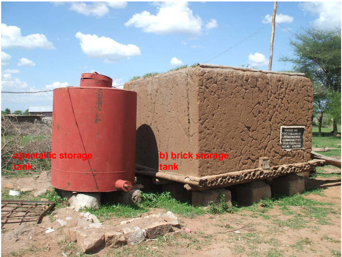
Plates 7: Peasant's (Mr. Lupande) grain storage tank at Senani. Above; a) on the left is a metallic storage; while, b) is a brick made grain storage.
