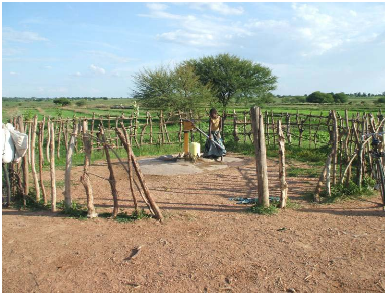
Plate 9: Health Sanitation Water (HESAWA) shallow wells under Sungusungu protection. The fence prevents animals trespass at Malemve, Kwimba district.
